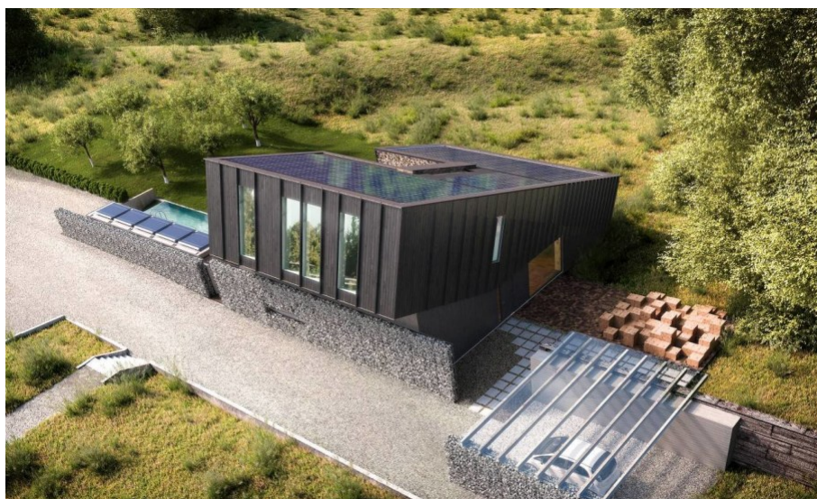
Ilustración 2: ZEB Pilot House: Casa con paneles solares. Recuperado de: http://bestdesignideas.com/zeb-pilot-house-an-interesting-energy-efficient-house
